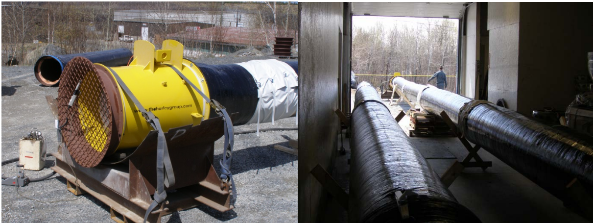
Figure 2 Fan duct assembly at HVT facility
