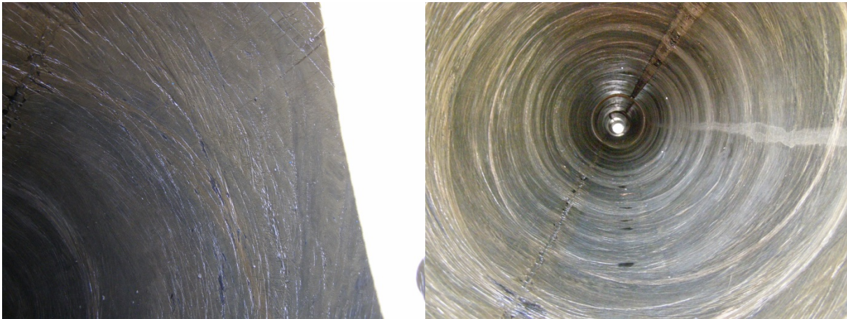
Figure 4 Internal surface of old style manufacture duct
