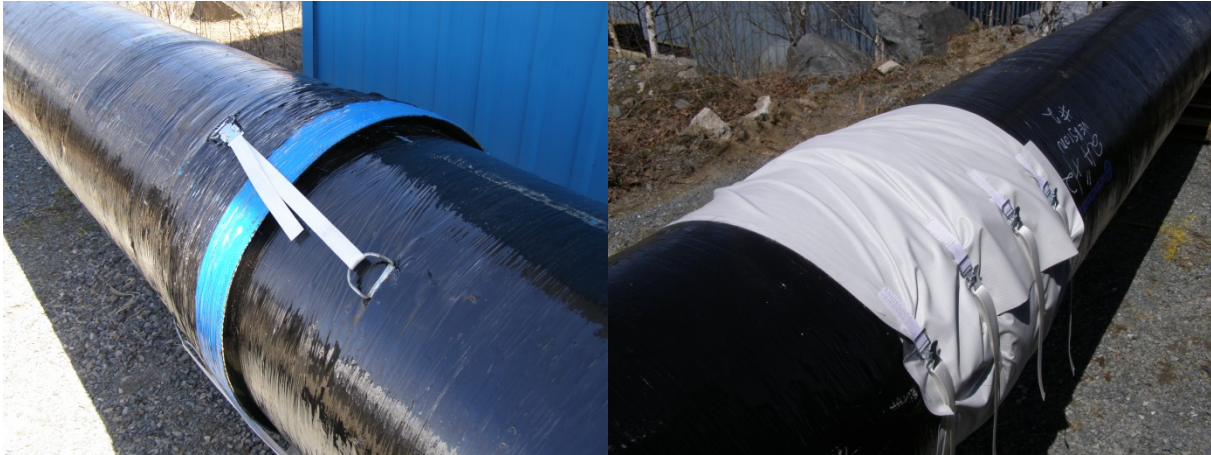
Figure 3 Jointing between two duct sections and optional wrap
