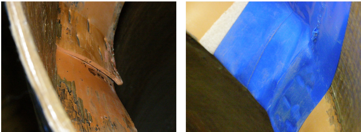
Figure 6 Photo of seal ( Left: original gasket; Right: patched gasket)
